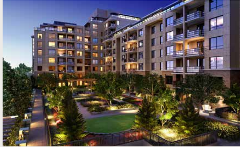
BRIDGELAND CROSSINGS Calgary, AB
